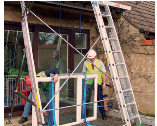
Attaching the new window
