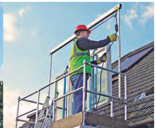
Hoisting to final position
