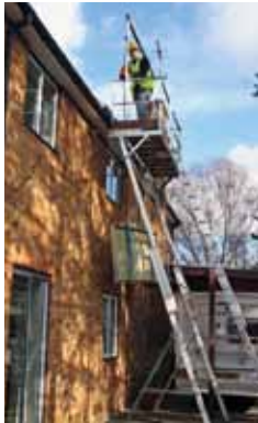
Hoisting to height
